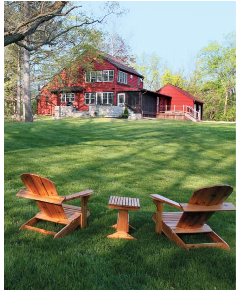
ABOVE: This renovation of a vernacular Michigan farmhouse is reminiscent of the Swedish red farmhouses depicted in the illustrations of artist Carl Larsson. Photograph by Howard Doughty
