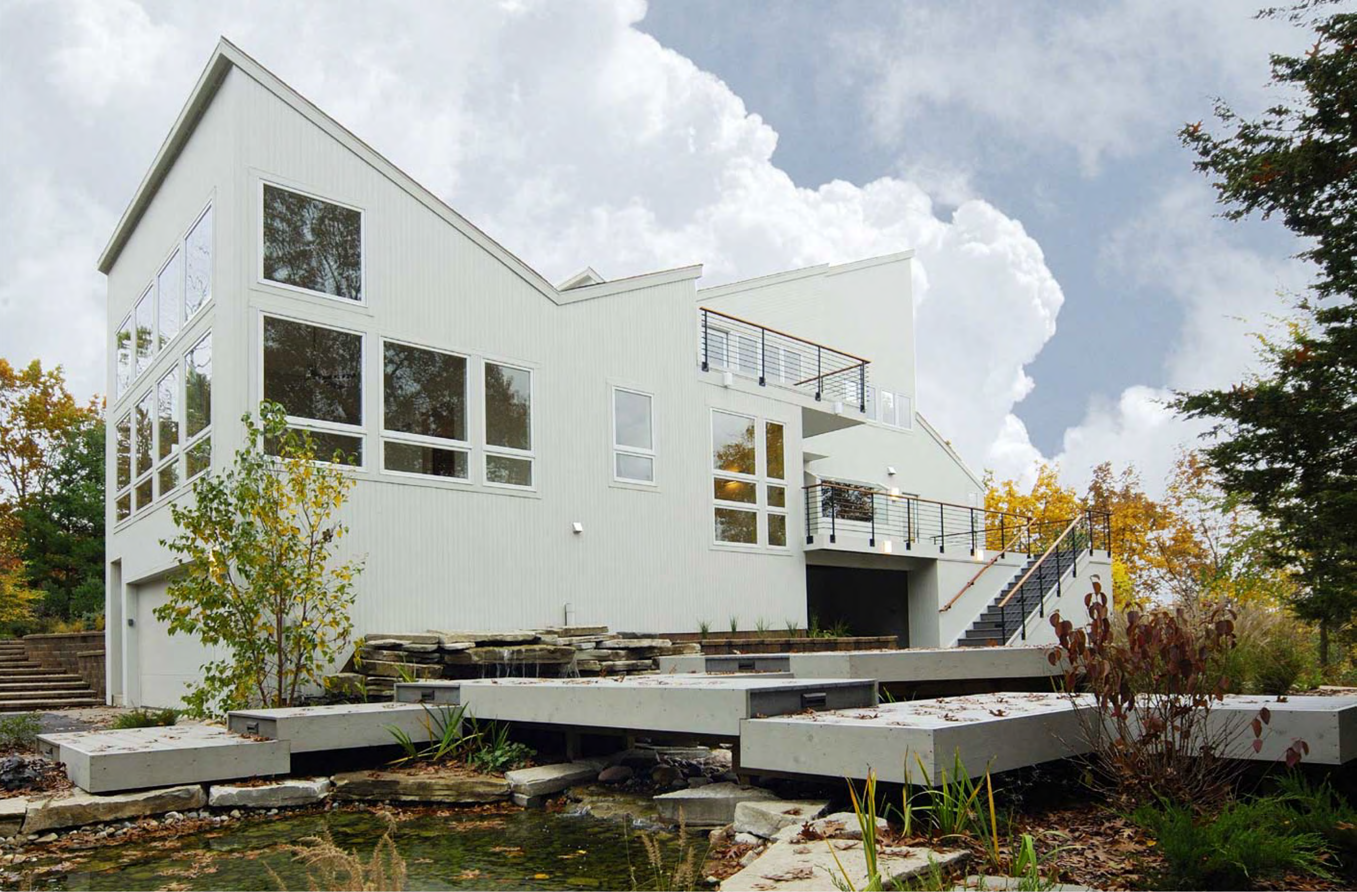
RIGHT: The winged roof angles crown the hilltop house and give the home a commanding presence. We used an inverted-pitched roof within the exercise room to allow for tall windows and a high ceiling within, focusing views to the outdoors. Working with Terrafirma Inc on landscaping and construction, we created an unforgettable home. Exterior deck platforms below compose a dynamic path through a pond and stream, offering a geometrically constructed base to the house within the larger natural setting.
